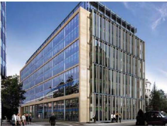
Basinghall Street is being developed into the global headquarters for Standard Chartered Bank, providing 200,000 sq ft.
